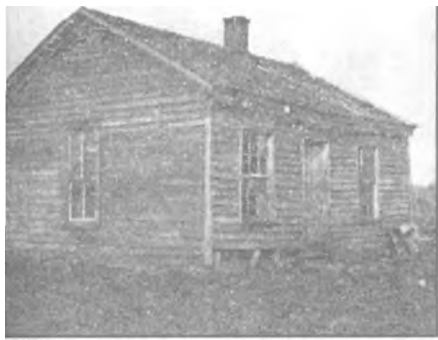
Mill Creek Church in Marion County was erected in 1855. courtesy of Don Porter
